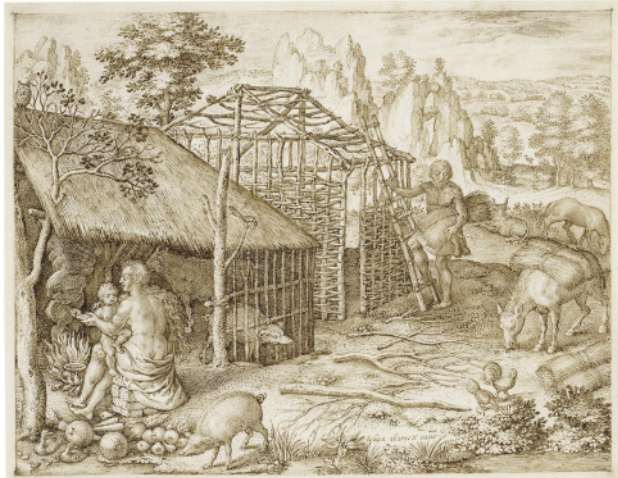
26 (11). Adam building a house
